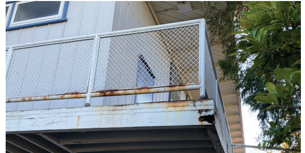
Deteriorating, rusting railings at Green Hills Elementary School.
