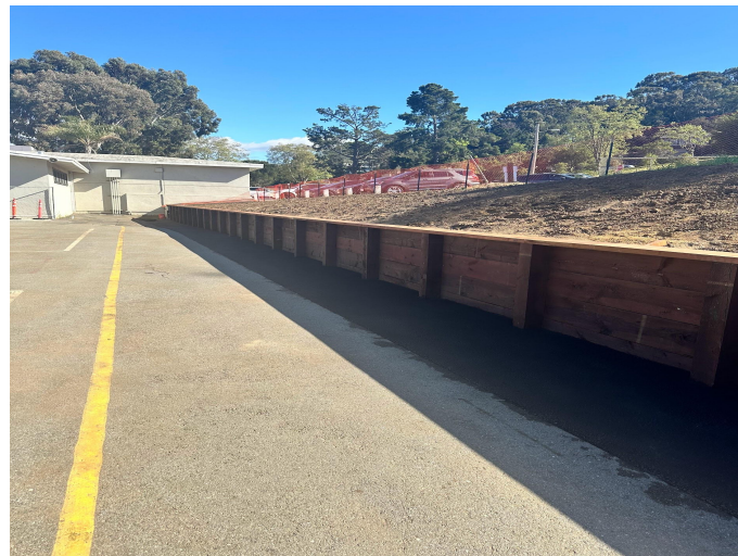
New Retaining Wall
